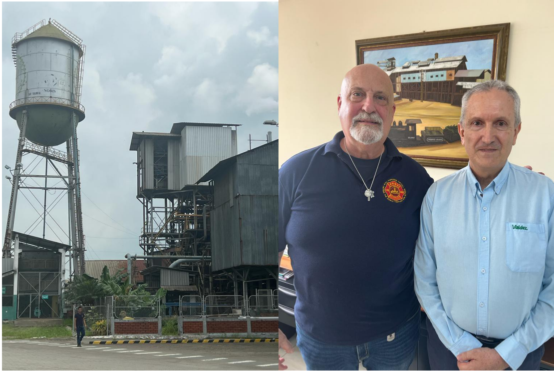
The Valdez Sugar processing plant with the original water tower still in operation left. Vince Forras and General Manager of Valdez Plant Carlos Valdivieso.
